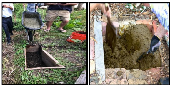
Fig: Filling of the pit with the cow dung slurry with mixture of other ingredients
