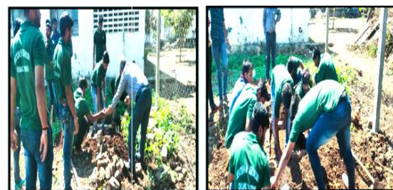
Fig: Making of pit of the CPP by Module Students (RBCA, Wardha)
